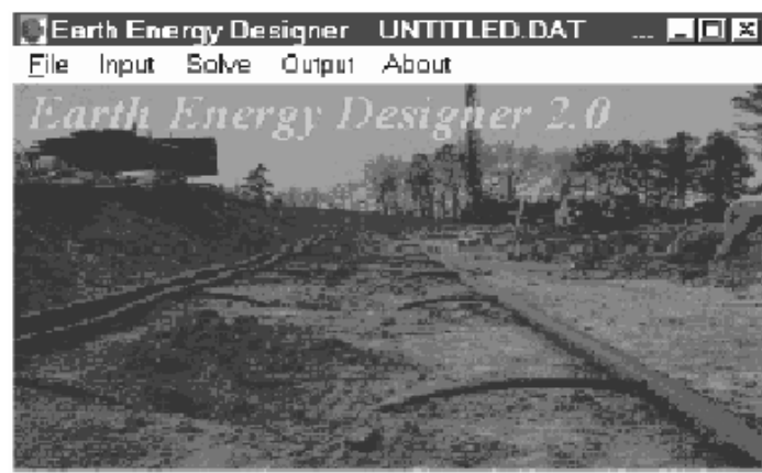
Fig. 2: Start screen of EED 2.0 (the photo shows the pipe connections of the 400-BHE-field at Richard Stockton College, New Jersey)
